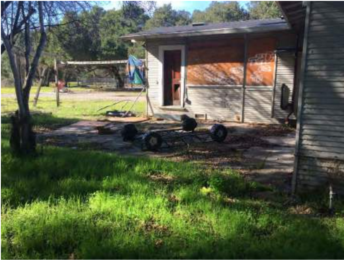
REAR OF HOUSE AT 1500 CAPITOLA ROAD
