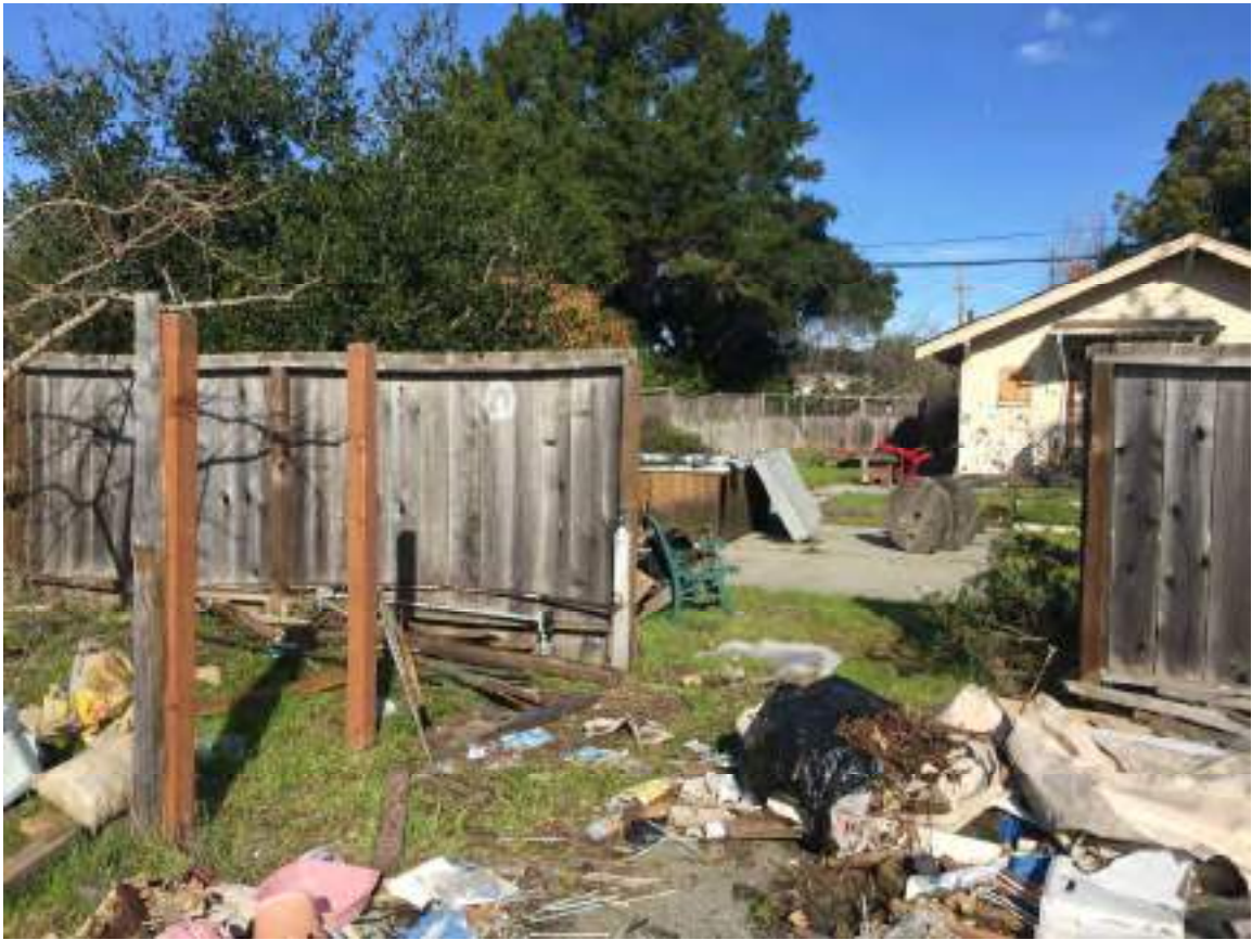
REAR OF HOUSE AT 1438 CAPITOLA ROAD
