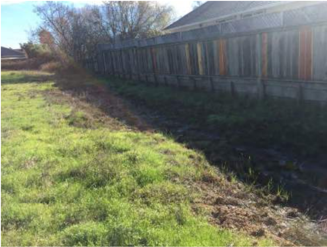
AREA OF STANDING WATER ALONG SOUTHERN BOUNDARY OF PROPERTY
