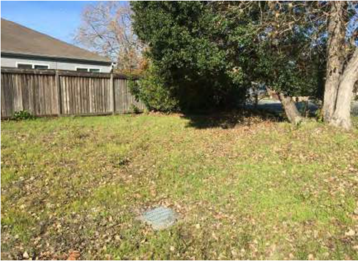
STORM DRAIN NORTHWEST CORNER OF 1412 CAPITOLA ROAD
