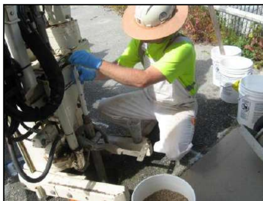
Shallow soil vapor probe installation via GeoProbe drill rig
