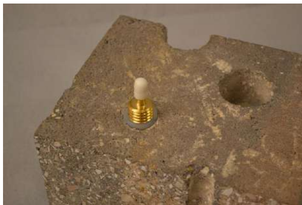
Figure 3. Installed Vapor Pin™
