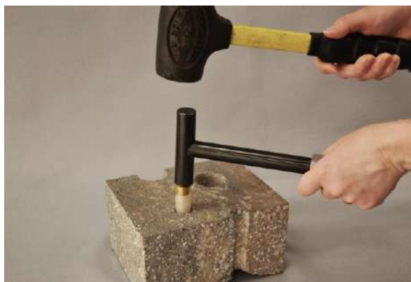
Figure 2. Installing the Vapor Pin™.
